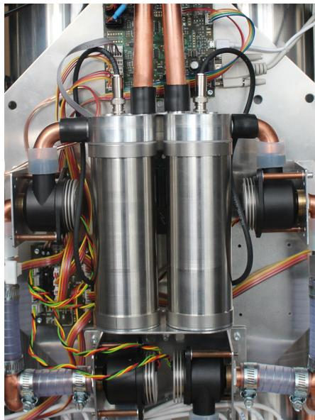
2. Disconnect and remove the tube going up into the charger filter unit. Disconnect the high voltage plug.
